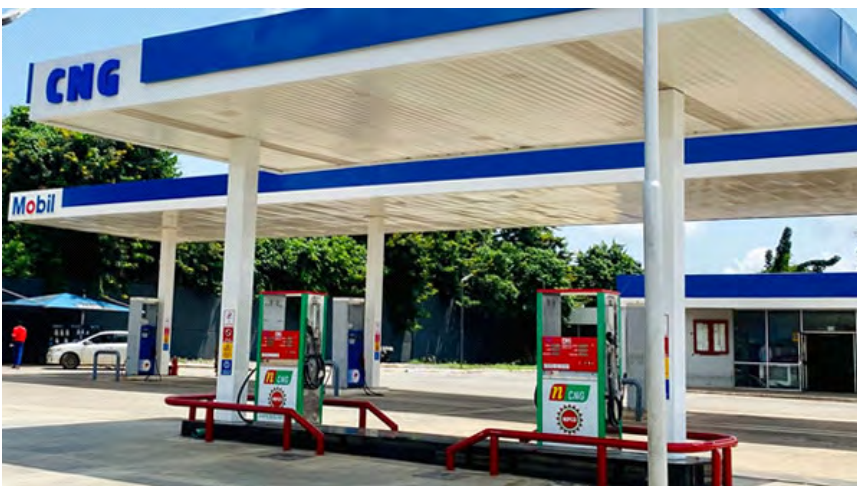
A CNG Service Station
